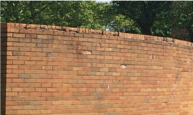
Spalling brick
