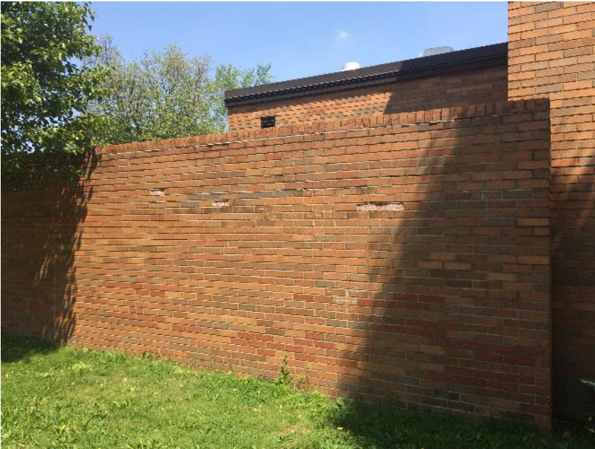
Spalling brick
