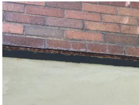
Rusted/delaminated lintel
